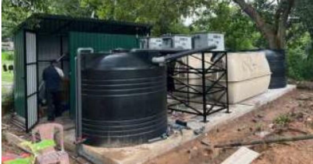
Pilot Johkasou Installed in Sri Lanka Institute of Information Technology (SLIIT is established in 1999)
