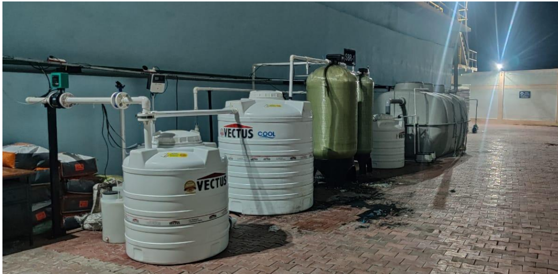
Pilot Johkasou Installed in the Indian Institute of Technology (IIT) Roorkee (IIT-Roorkee is established in 1847, the oldest technical institution in India)
